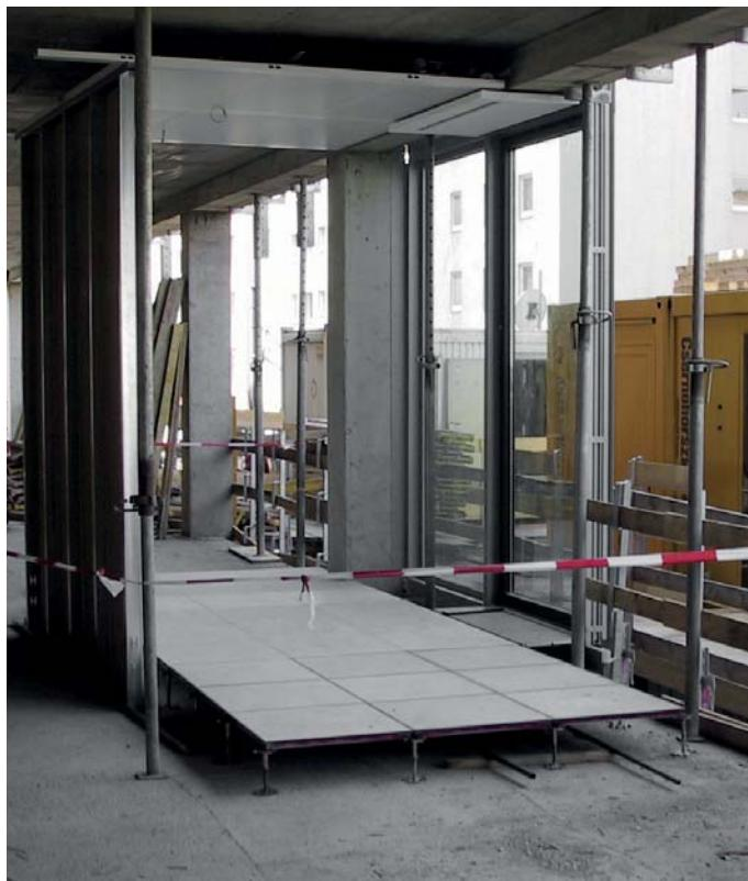
Example of double floor structure installation
